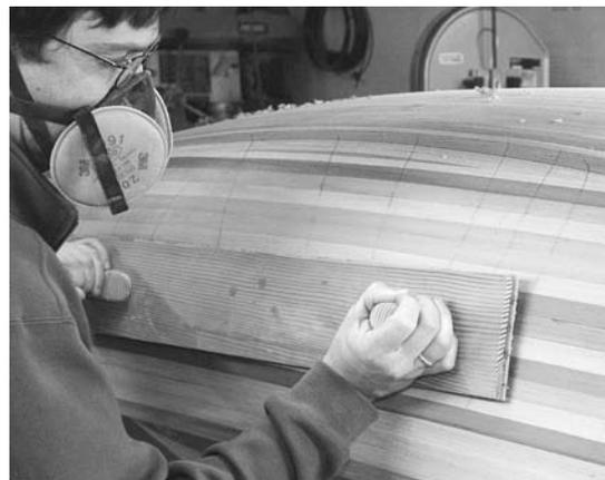
**Figure 7-8.** By working until all the pencil marks are gone you will be sure the whole surface has been sanded and is quite fair. This fairing process can be done with very coarse sandpaper such as 40- or 60-grit. Try to sand with the grain to minimize the scratches.
