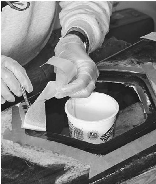
Cut the hatch lip with an inner diameter about  $\frac{3}{4}$  inch smaller than the hole and with the same outer shape as the spacer. Glue the lip in place. After the glue has set, apply a fillet of dookie schmutz around the outer perimeter and glass the underside of the hatch.
