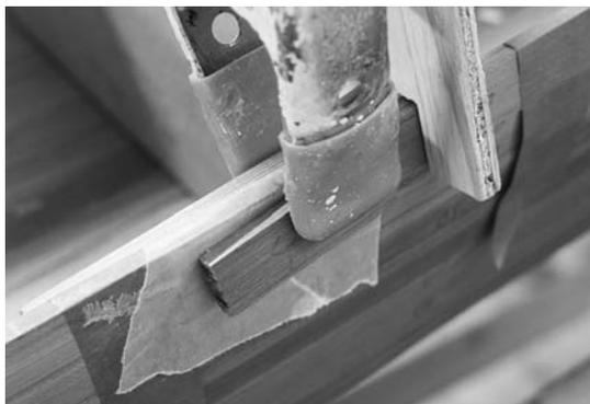
**Figure 13-22.** Butt together the strips cut with the miter box in place on the boat while stripping. Use waxed paper so the scrap strip used to help align the joint does not stick to the boat. Put masking tape on either side of the joint to hold the strips in place relative to the strip below.
