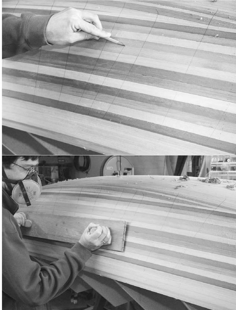
**Figure 11-17.** To get a fair, consistent surface you want to sand everything to approximately the same degree. You can provide sanding guides by scribbling on the surface with a soft pencil. Do not press hard, and use the side of the pencil point so you don't create grooves in the wood.
