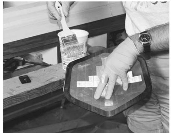
**Figure 13-72.** The edges of the hatch covers are covered with 2-ounce fiberglass cloth and then a couple of layers of epoxy. Making a handle out of tape makes it easier to hold onto the piece as you work.
