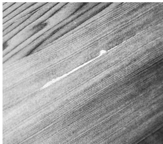
**Figure 7-16.** If there is any glue left on the surface, it should show up when you wet the boat with water. Carpenter's glue shows up white when it is wet. Other waterproof glues would not show up as easily. You can usually scrape off the glue, let the wood dry, and then give the region a thorough sanding. Mark the area with a flag of tape so you can find the spot again after the wood dries.
